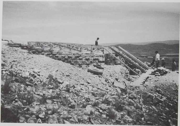
EARTHSHIP AT 1,400 FEET IN BOLIVIA SHOWING THE DIFFERENT GREENHOUSE ANGLE FOR THE HIGHER SUN NEAR THE EQUATOR
