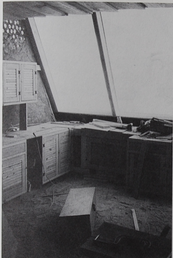
SOLAR OVEN UNDER CONSTRUCTION
