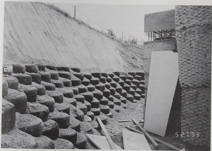
TIRE RETAINING WALL BEHIND EARTHSHIP IN JAPAN.
