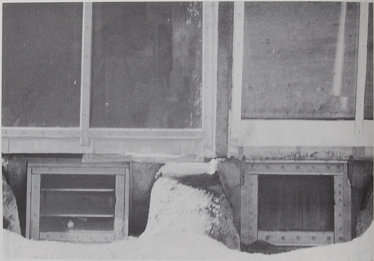
SOLAR OVEN AND TOILET INSTALLATION UNDER CONSTRUCTION
