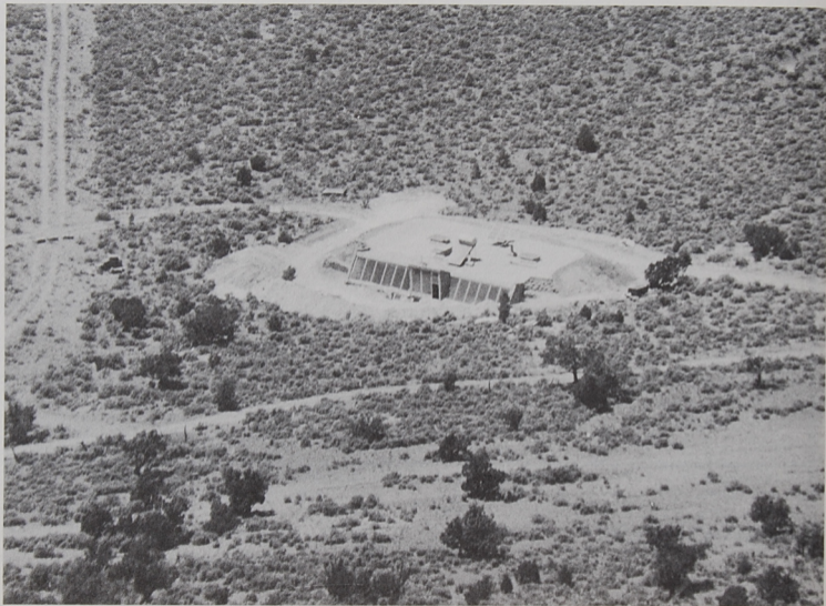
GENERIC EARTHSHIP AT S.T.A.R. UNDER CONSTRUCTION
